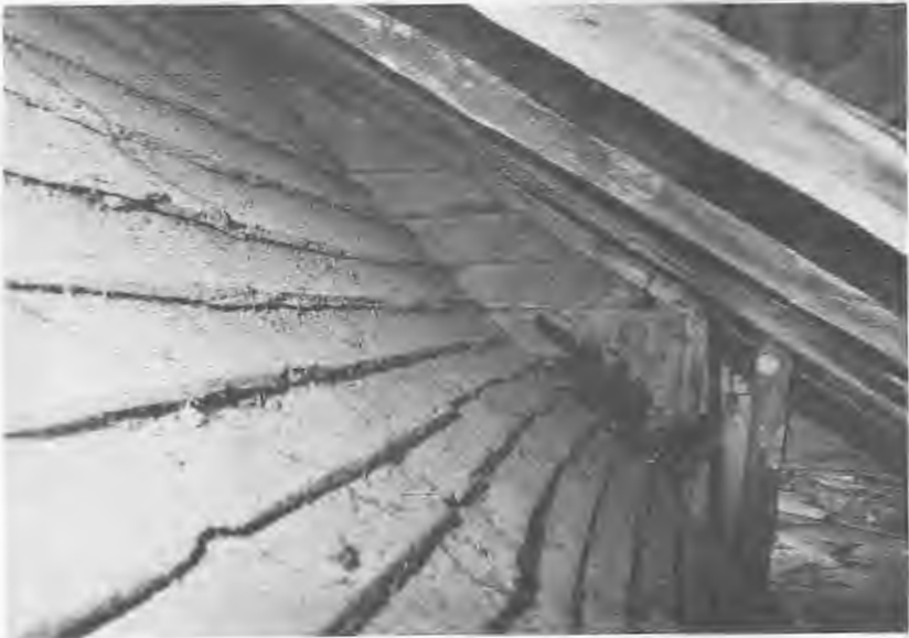
Clapboard roof showing protective roof built around it
